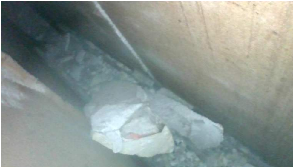
Figure 3- Demising Wall Borescope
